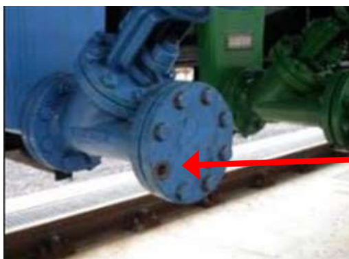
Figure 5: flange system with missing bolt.
